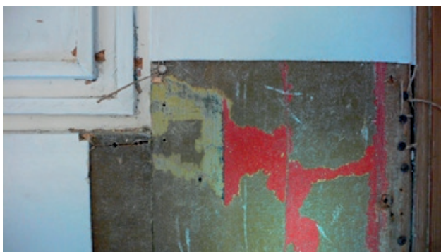
Fig. 6 North wall of the Withdrawing Room. Detail of the surface of the discoloured varnished patent yellow scheme (Decoration 7 c.1810) under hessian. Areas of the red frame and black lining of Decorations 3 and 4 have been exposed.
