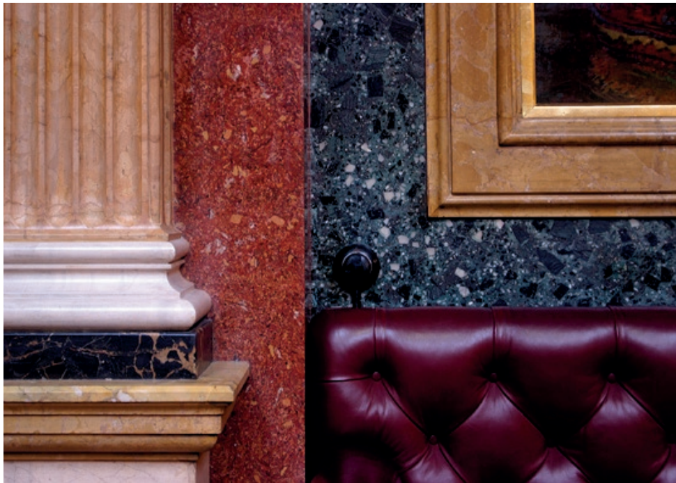
Fig. 5 Detail of the scagliola finishes on the colonnade walls.
